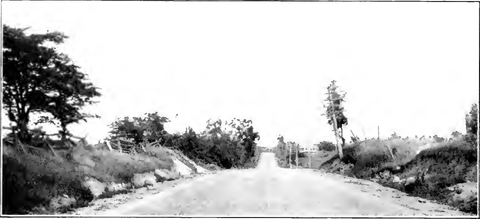
HAMILTON-KITCHENER PROVINCIAL HIGHWAY Asphaltic concrete pavement 20 feet wide south of Galt.
